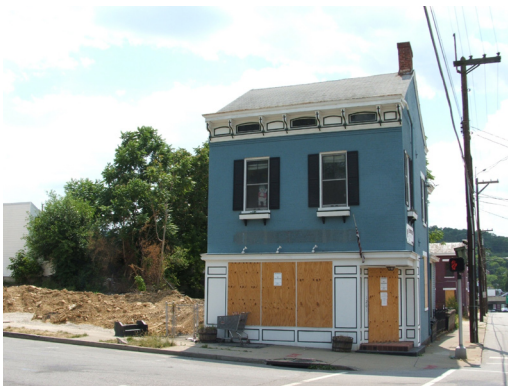
Picture of Flannery Painting Building on 12 th Street proposed to be relocated.
