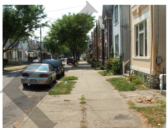
Sidewalk along Woodburn Avenue
