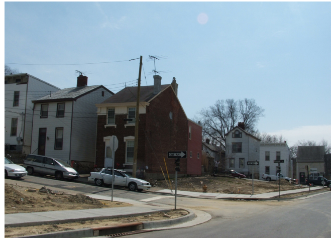
Current structures along the St. Elizabeth Medical Center Covington access road
