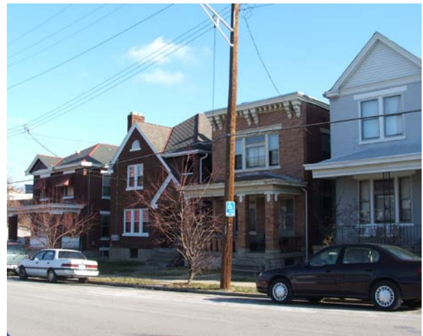
Existing homes north of 12 th Street and east of Main Street
