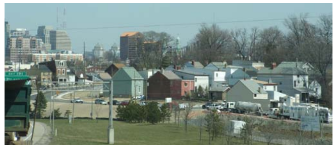
New access road off of Main Street to St. Elisabeth site
