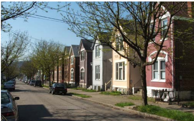
Woodburn Street south of Linden Street
