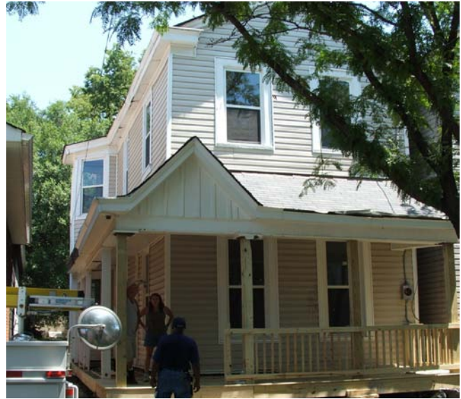
Rehabilitation of home within the Study Area
