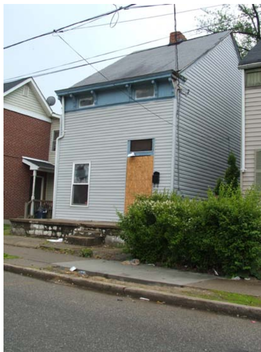
House in poor condition
