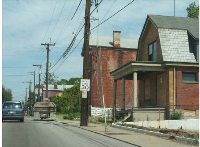
Homes on the south side of 12 th Street prior to demolition
