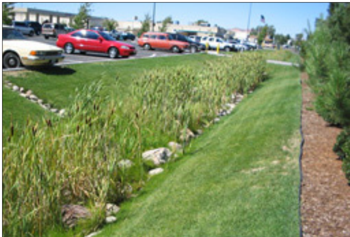
Figure 14: Retention pond and rain garden
