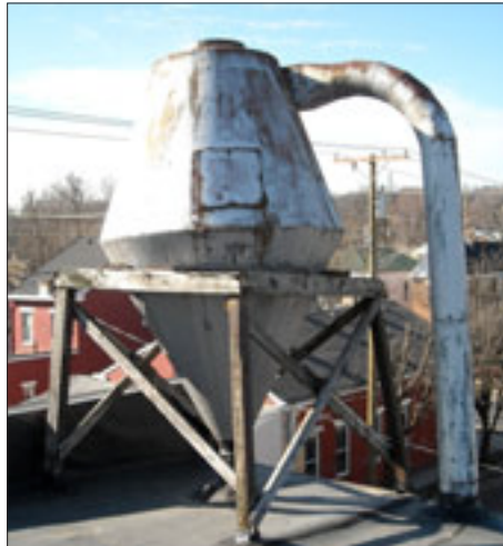
Manufacturing elements that were used historically add interest to the building fabric. These elements should be retained when feasible.
