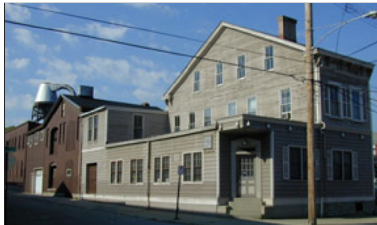
An assembly of building forms, materials and heights make up this interesting building complex. Note most of the building forms reflect individual building form, mass and scale of buildings found within the area.
