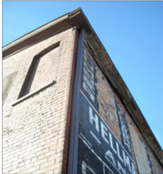
Hand painted signs are character-defining features on warehouse buildings.
