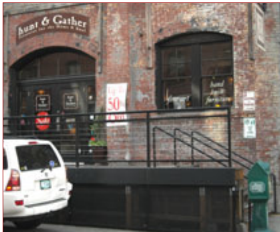
The handrails shown here are appropriately installed on a loading dock. The railing remains transparent allowing one to see through to the historic building fabric.
