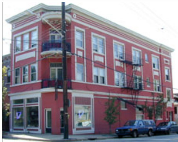
A three story building with a commercial storefront anchors this corner. Note the doors in this building were inappropriately altered.
