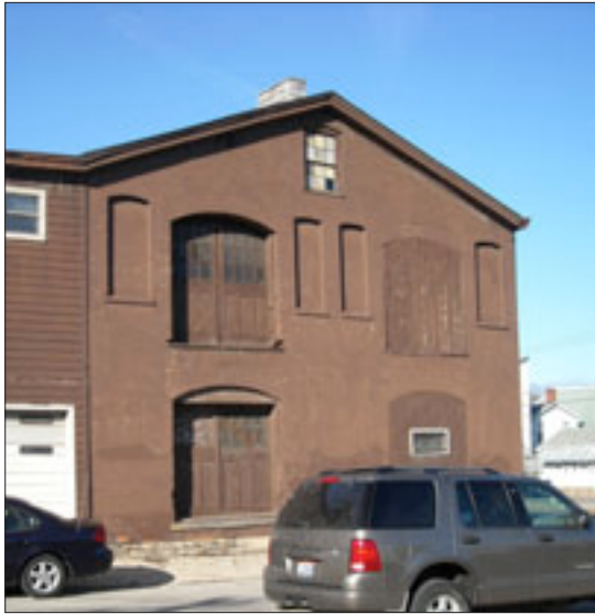
Large oversized doors were used historically for loading and materials. Today, these could be re-used for the same purpose or a new adaptive reuse could be employed.
