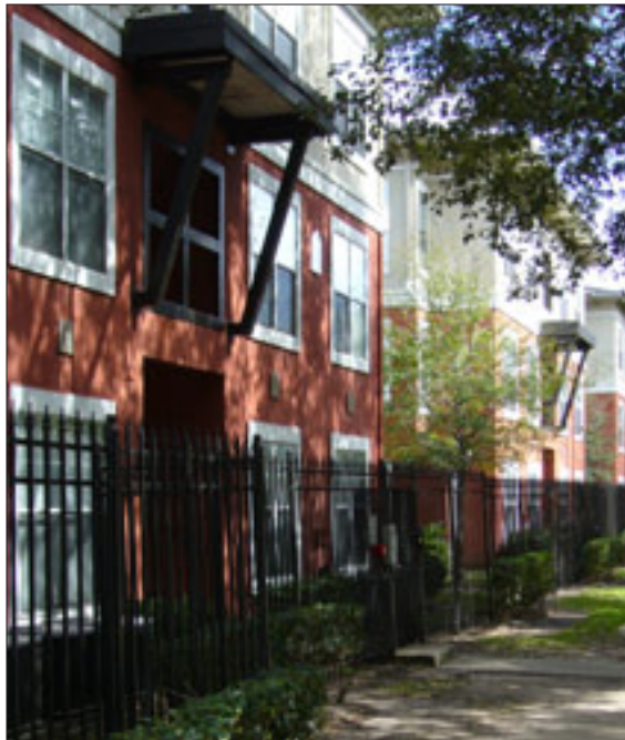
A new design that draws upon the fundamental similarities among older buildings in the area without copying them is preferred.
