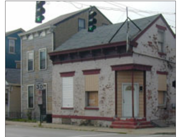
Corner buildings with recessed corner entries were common. This entry was inappropriately modified.
