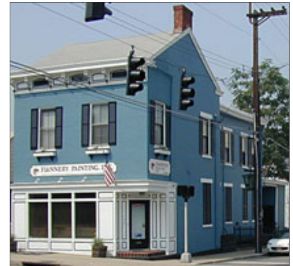
Italianate Style (two story, corner commercial). Front elevation before the building was moved to its new location.
