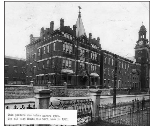
Stone piers supporting metal fences, as well as solid stone walls, were seen.
