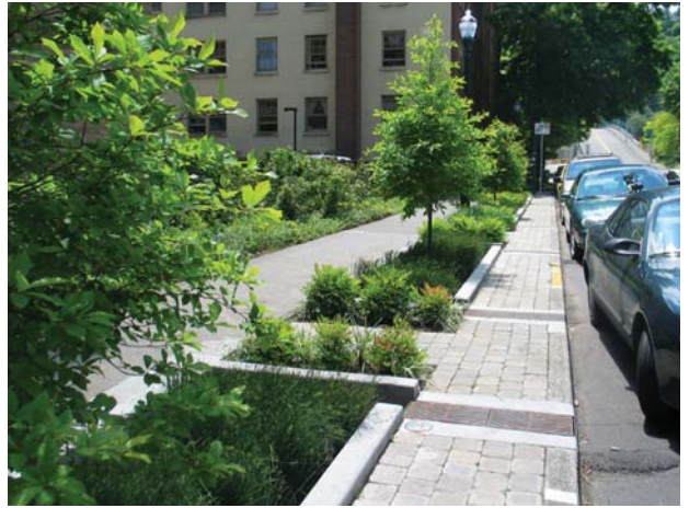
Figure 4.4.3: Stormwater Planter Box
