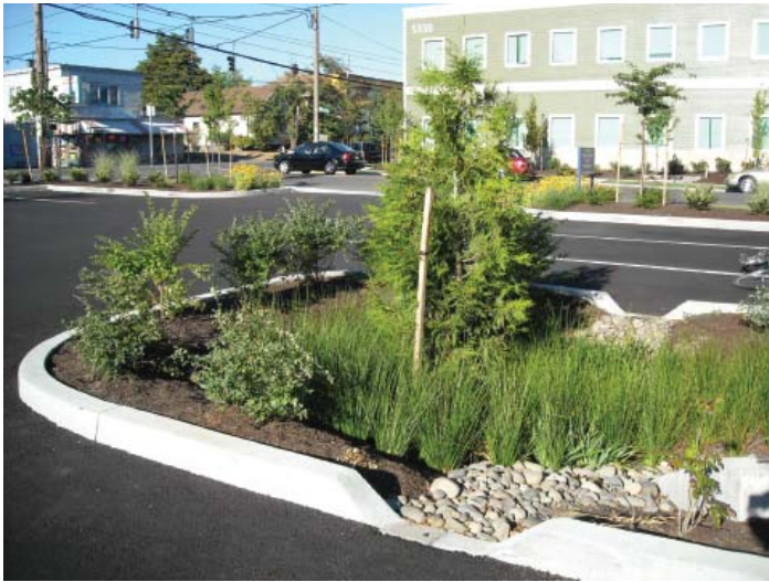
FIGURE 6.19 RAIN GARDEN/BIORETENTION AREA
