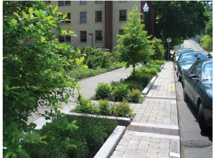
FIGURE 6.20 STORM WATER PLANTER BOXES
