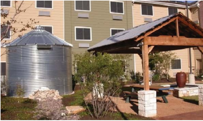
FIGURE 6.21 RAIN BARRELS AND CISTERNS
