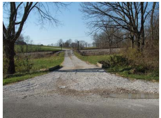
View of railroad crossing
