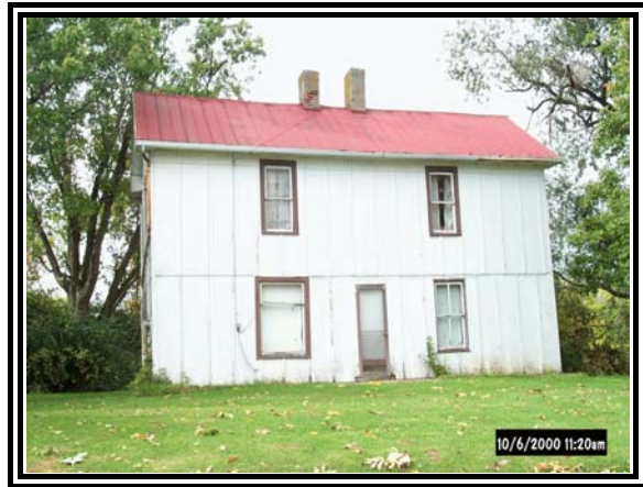
The preservation of distinctive historic architecture such as this board-and-batten house at 751 Stephens Road (KE-TM-5) should always be part of the planning process.
