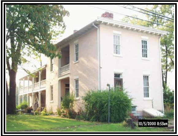
The Oxley House at Independence (KE-I-9) is one of the finest historic residential properties outside the Kenton County Ohio River communities.
