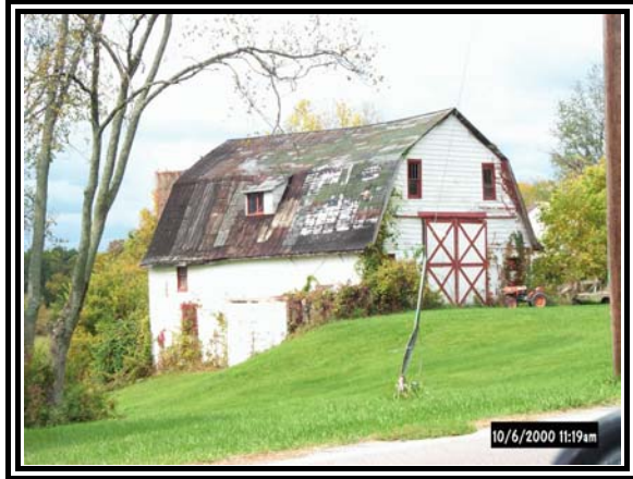
Agricultural outbuildings such as this dairy barn on Stephens Road (KE-TM-4) provide important reminders of Kenton County's former agrarian character.
