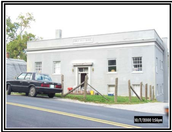
Although significantly altered from its original appearance, the Forest Hills School (KE-TM-13) is nonetheless an important component in Kenton County’s educational history.
