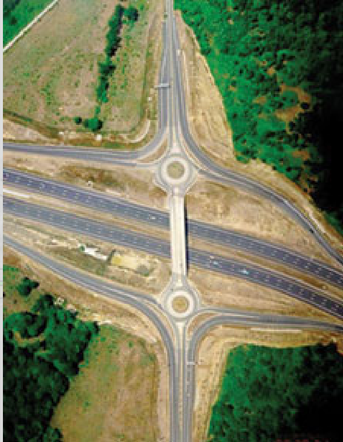
Maryland State Highway Administration
