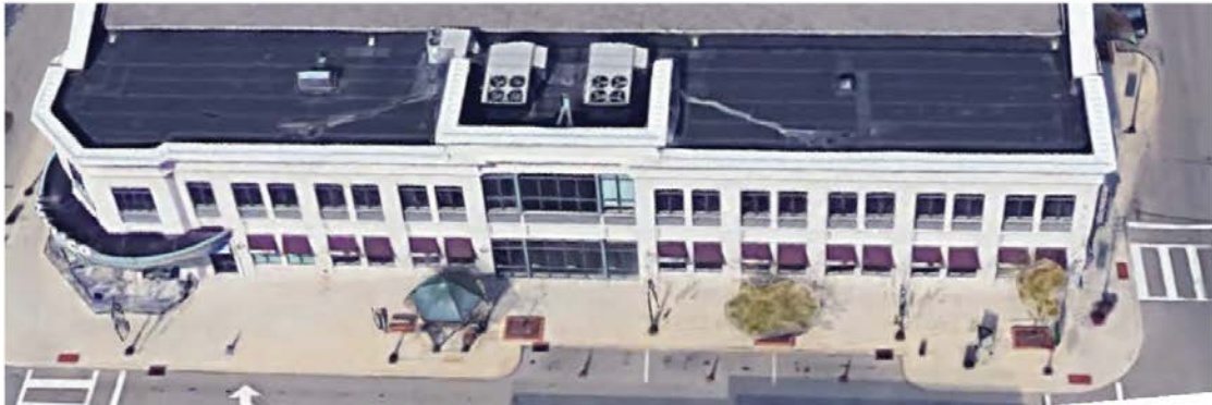
Figure 10.16.4-44 Rooftop Utilities Screened from the Public Way by a Parapet
