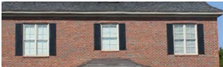
Inappropriately Scaled Shutters: Not Permitted
