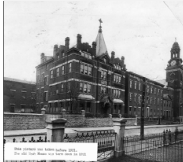
Stone piers supporting metal fences, as well as solid stone walls, were seen.
