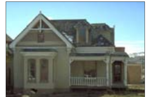
The same house as above, preparing to be lifted from its foundation
