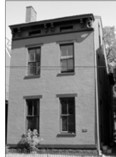
Roof cornices and stone lintels above the windows are typical features.
