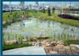
4 STORMWATER FILTRATION STORAGE CELL
