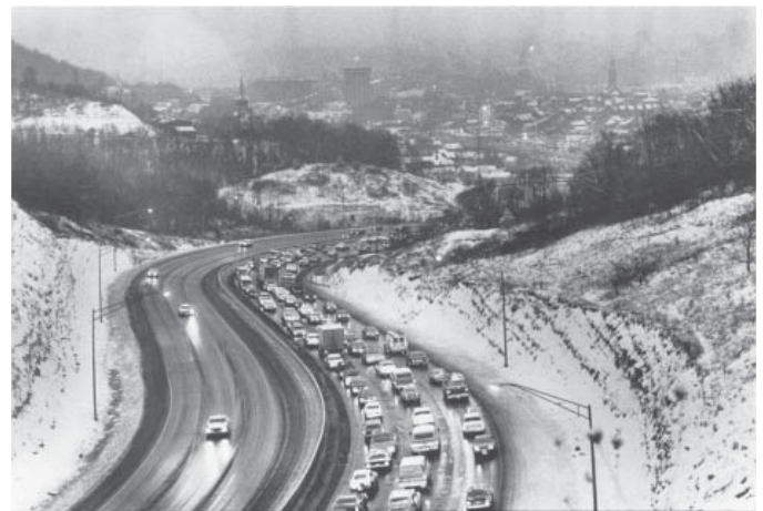
Figure 2.1 "The cut in the hill" on I-75, looking north toward Cincinnati. (Courtesy: Kenton County Library) This undated photo shows a historical condition on I-75.
