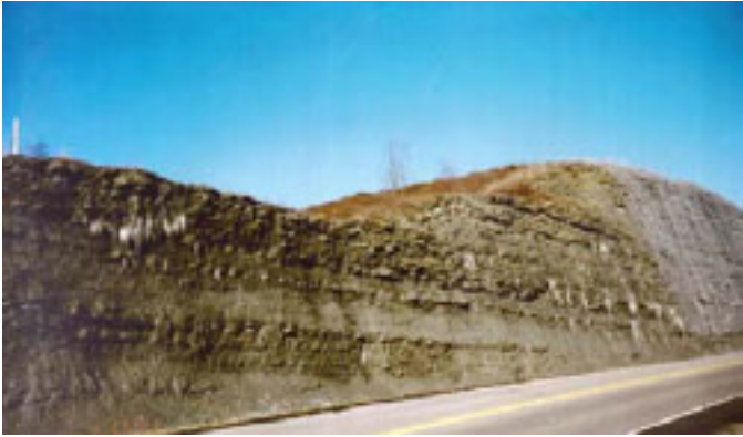
Figure 3.7 Exposed Kope geology along a road-cut.
