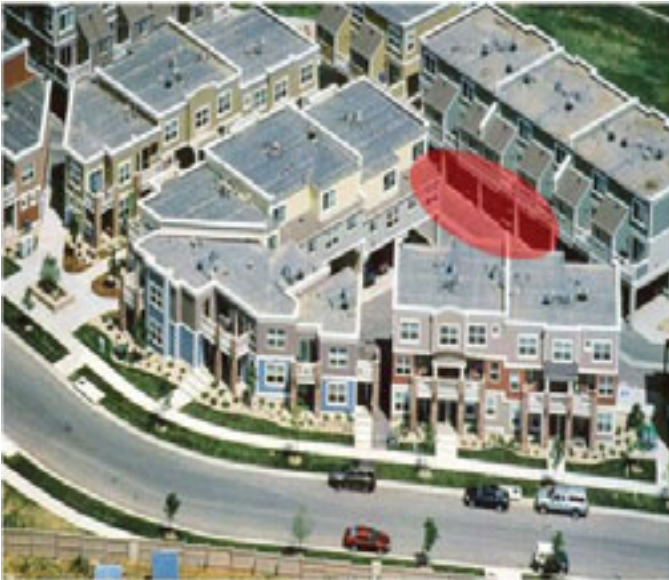
Figure 6.7 An example of a “tuck under” parking lot (highlighted in red) where parking is placed partially under a building.
