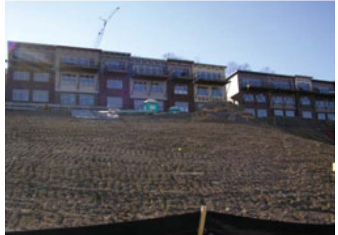
Figure 3.10 Hillside development in Northern Kentucky.
