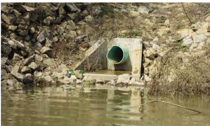
Figure 4.2 – Combined Sewer Overflow
