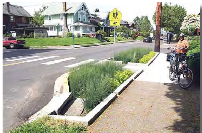
Figure 4.3 – Example of vegetated curb extension that captures stormwater before entering the storm sewer.
