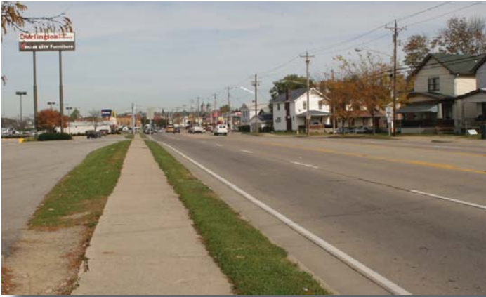
Figure 8.1 - Sidewalk Along Winston Avenue
