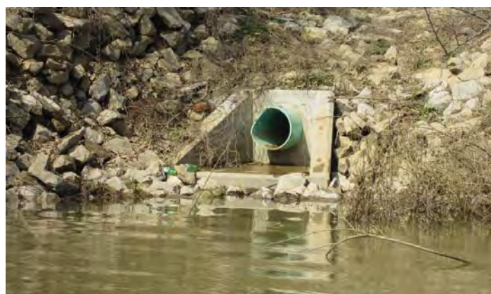
Figure 4.2 – Combined Sewer Overflow
