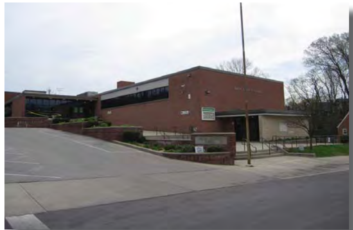
Figure 5.2 – Ninth District Elementary
