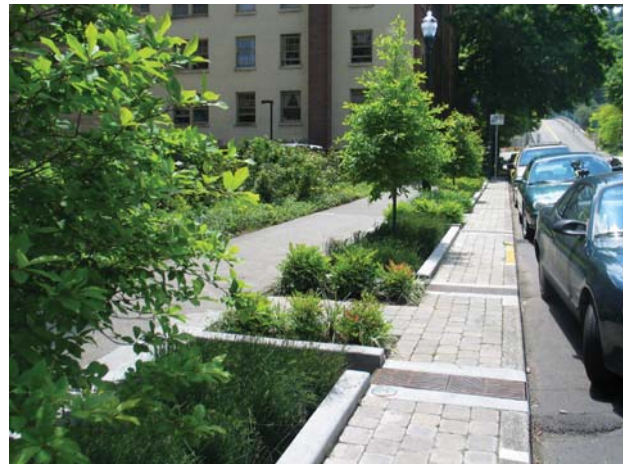
Figure 4.4.3: Stormwater Planter Box
