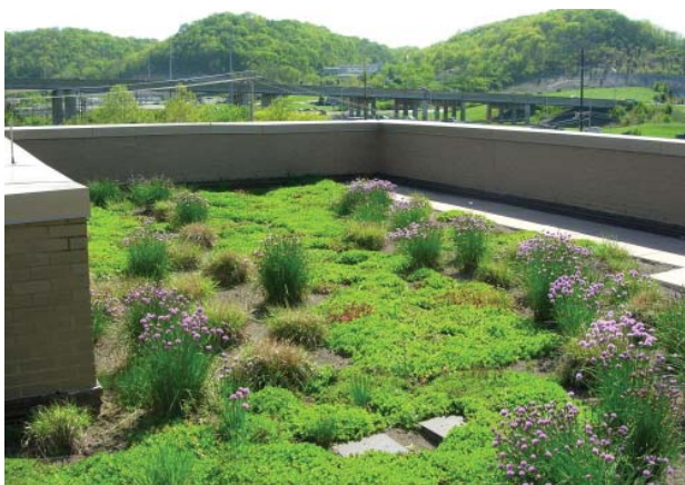
Figure 4.4.5: Green Roof in Use at SD1
