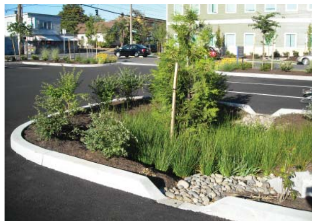
Figure 4.4.6: Rain Garden in a Parking Area
