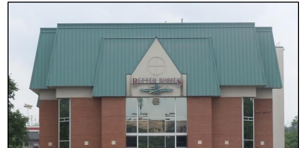
Above: The size and scale of mansard roofs overpower and detract from the character and form of a building or structure.
