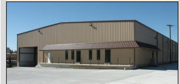
Above: Corrugated metal buildings project an isolating and sterile environment found in industrial areas and are not appropriate in a neighborhood or "main street" area.
