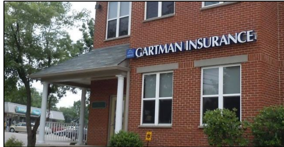
Above: The use of a simple recessed entry and porch feature help to break up a building façade and add character to a structure.
